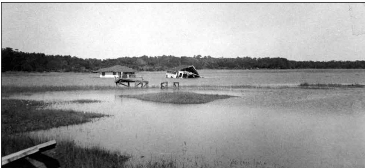
In 1954, Hurricane Hazel's tide was 11½ feet above mean sea level, and 10-foot-high waves pushed houses on the south end from the oceanfront and the Bird's Nest section to the middle of the salt marsh. Owners recovered their homes on the first full-moon high tide after Hazel by floating them out of the creek with cables and restoring them on their properties. These two are the Hiller Viller and the Michau house.
